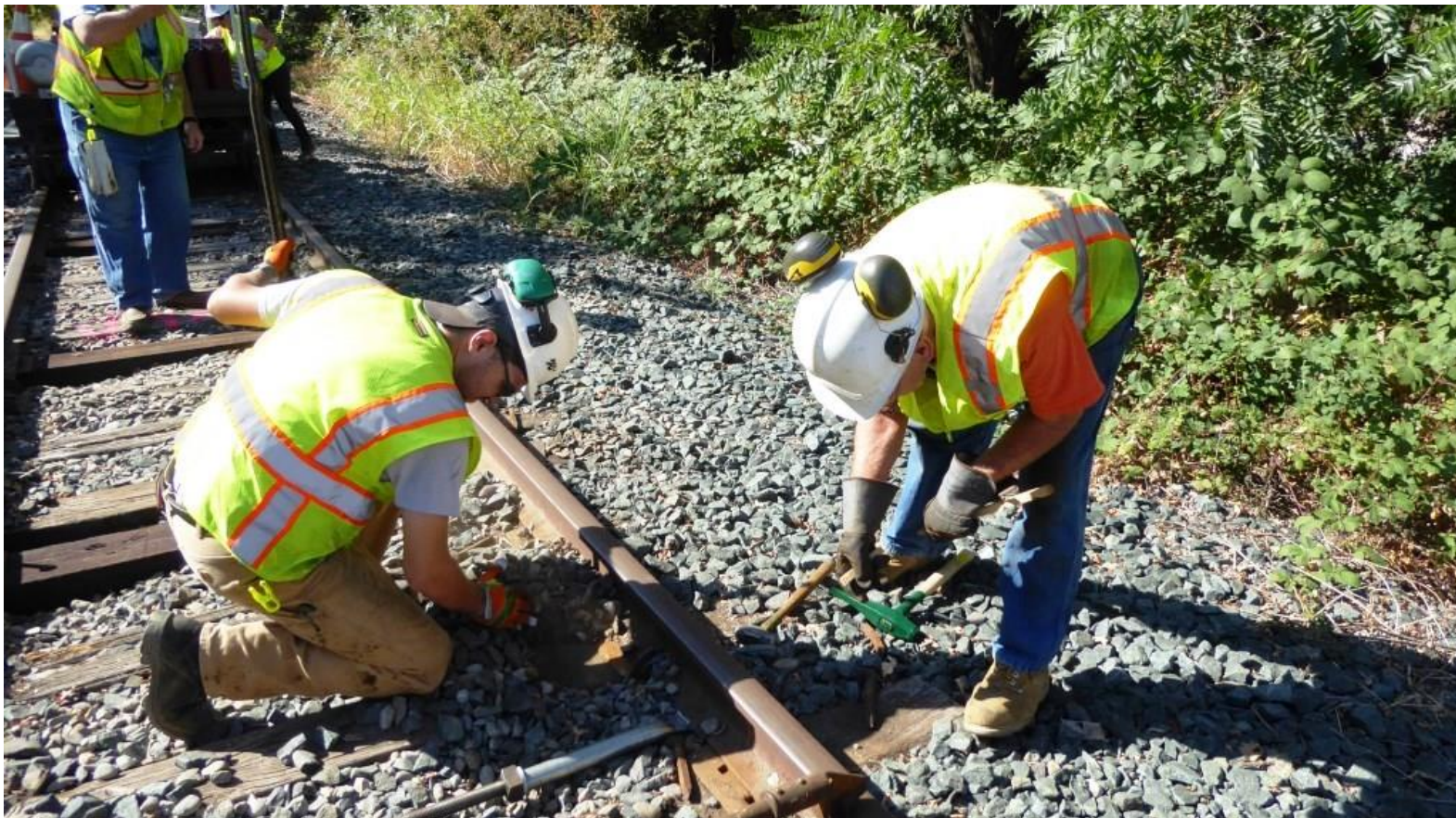
Kyle and Clem pull spikes and plug the old spike-holes
