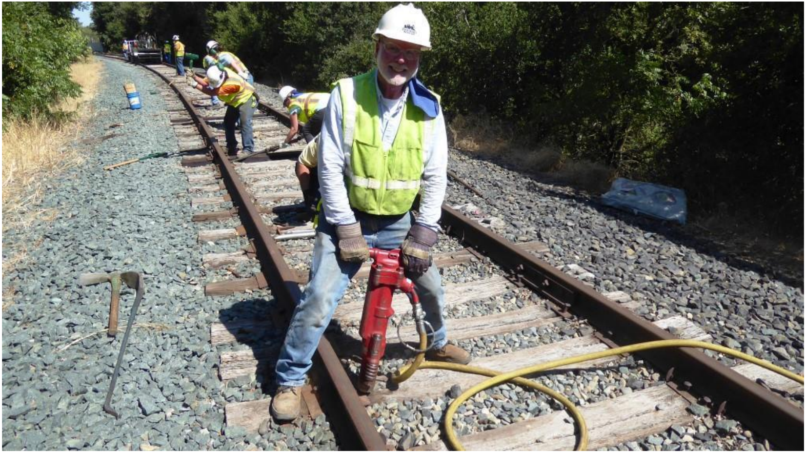
Mike M. is excited for some good ol' fashioned pneumatic spike-driving fun!
