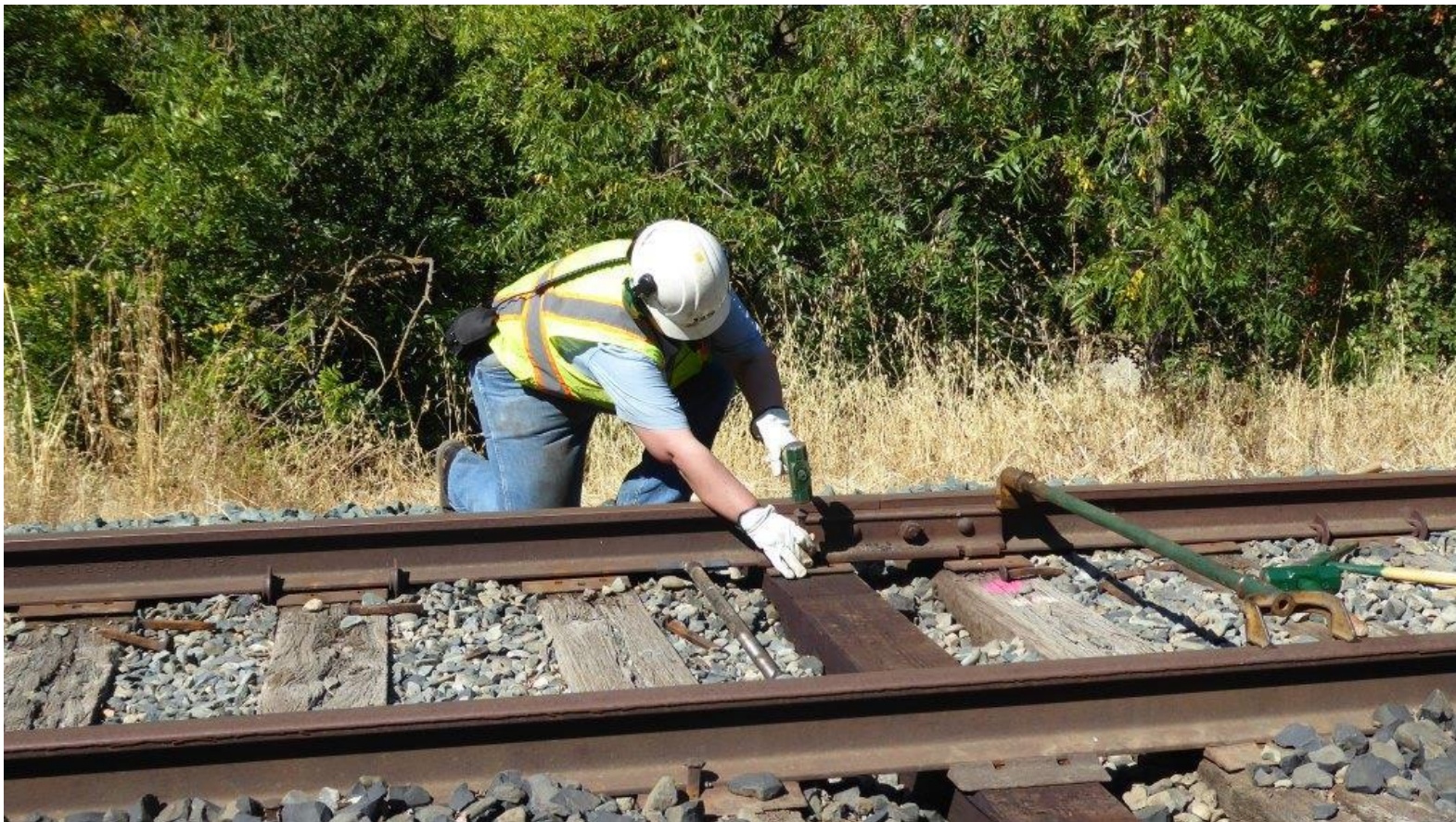
Heather sets spikes where the rail has been spread to the proper gauge.
