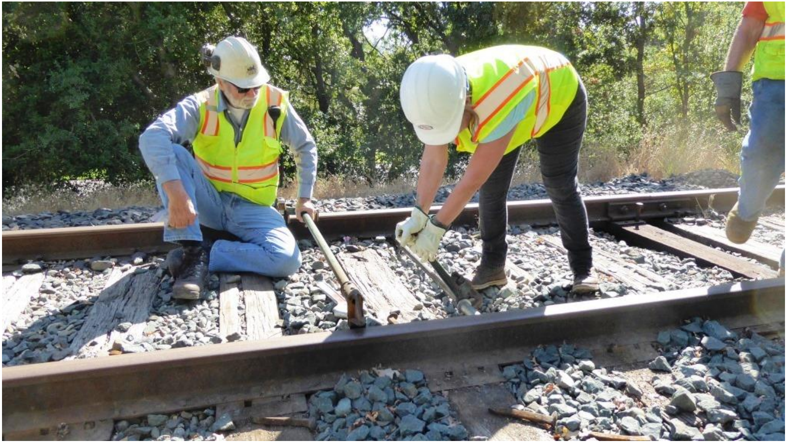
Alan and Mary set up the rail spreader
